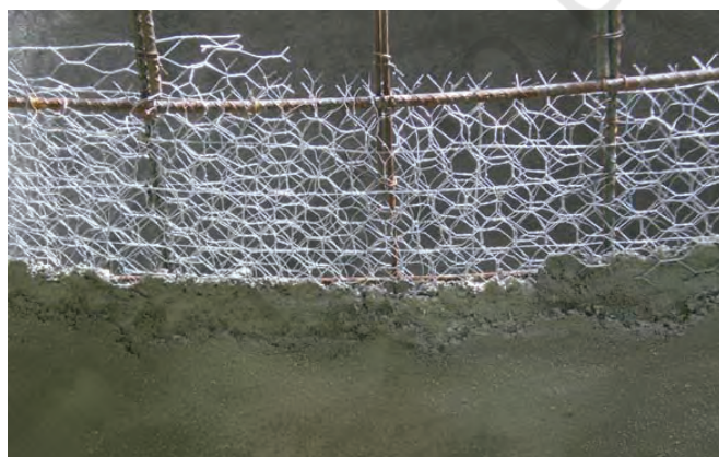
Fig.2.23: Ferro Cement work
