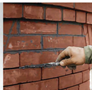
Fig.4.17: Raking needle
