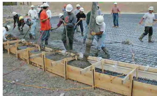
Fig.2.14:Reinforced Cement Concrete
