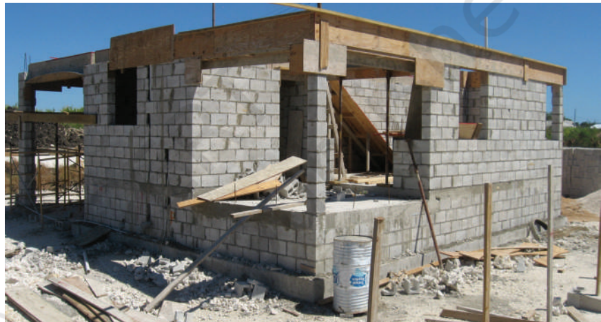
Fig. 4.12: Concrete block wall in house construction
