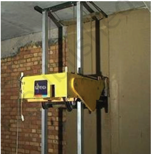
Fig. 3.2: Plastering with machine
