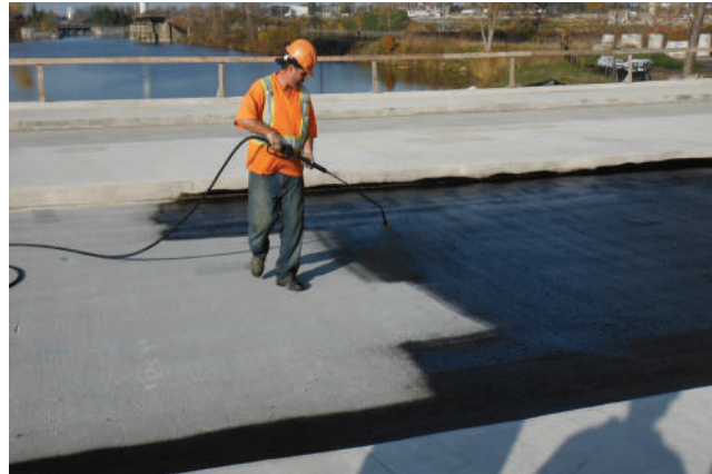
Fig. 5.9: Spraying waterproofing material
