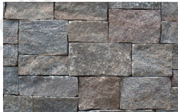
Fig. 1.18: Ashlar rock or quarry faced
