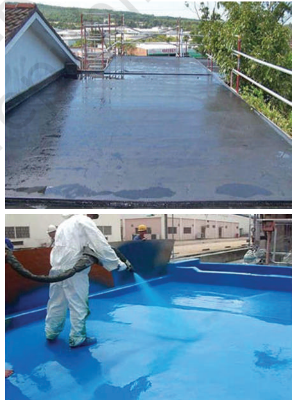
Fig. 5.17: Poly Acrylic chemical coating waterproofing
