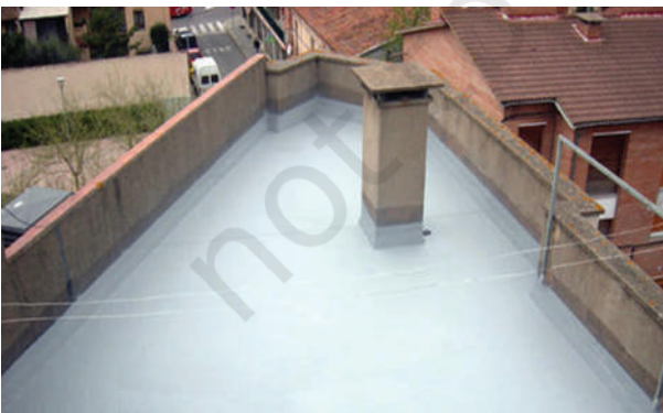
Fig. 5.15: Polyurethane Liquid Membrane
