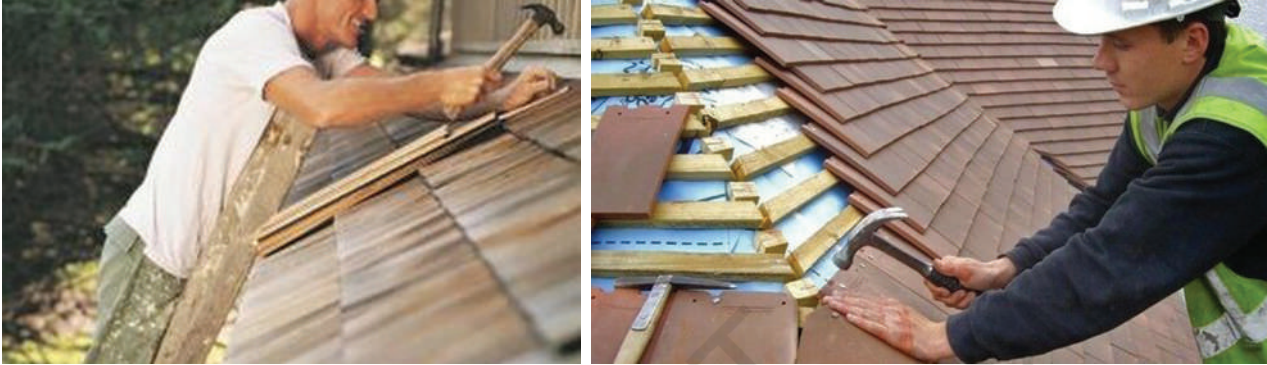
Fig. 5.18: Pre-monsoon roof repairing
