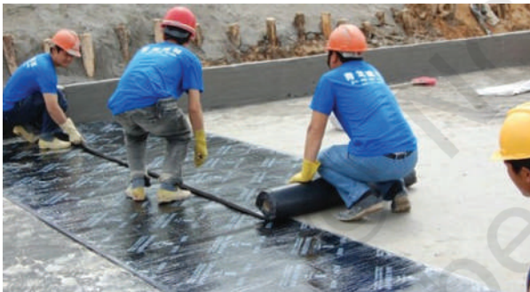
Fig. 5.14: Bituminous Membrane Laying
