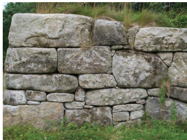
Fig. 1.12: Dry Rubble Masonry
