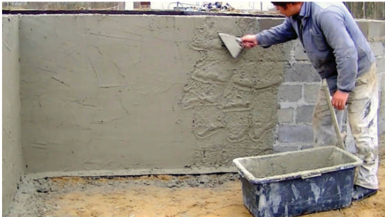
Fig. 3.3: Plastering with manual labour
