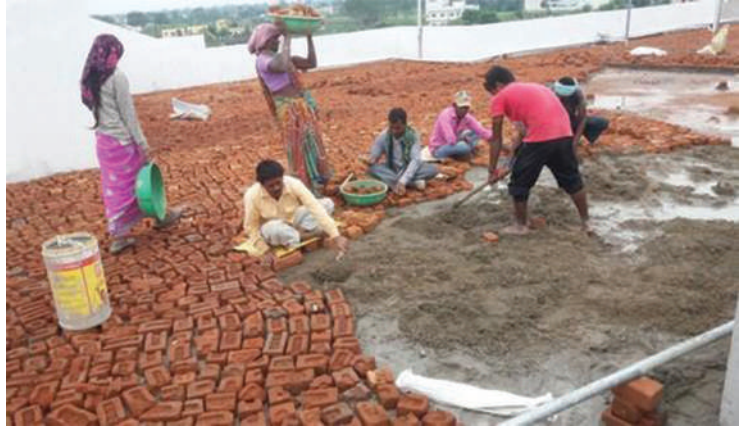
Fig. 5.16: Brick Bat coba waterproofing
