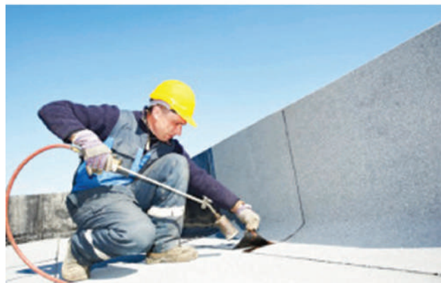
Fig. 5.2: Execution process of waterproofing works
