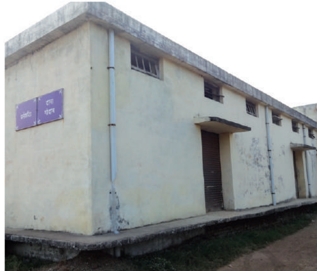
Fig. 4.15: Feed godown on raised platform
