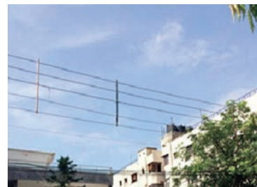
Fig. 4.18 Vertical Line Spacers
