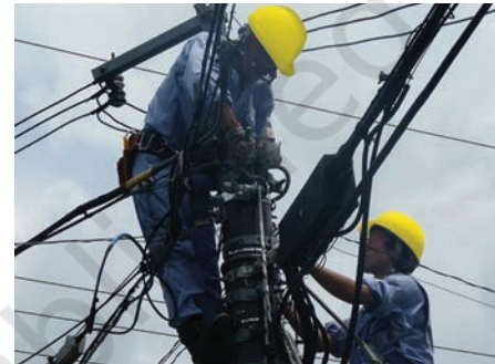
Fig. 4.53 Inspection of Power Distribution Lines
