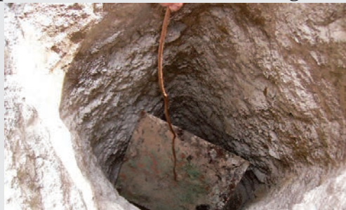
Fig. c: Placing a copper plate in the pit
