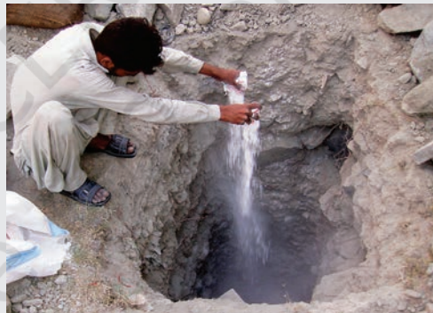
Fig. b: Filling the pit with coal and salt
