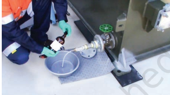
Fig. 11.22: Draining oil from a transformer
