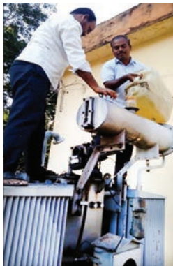
Fig. 11.20: Manual filling of oil in a transformer
