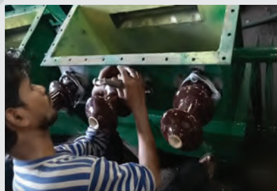
Fig. l: Fitting high voltage bushing on the transformer
