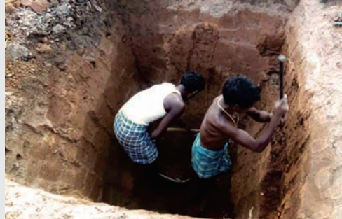
Fig. a: Excavation to form a pit for earthing
