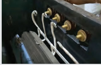
Fig. n: Assembly in the transformer tank
