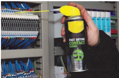
Fig. 11.7: Equipment cleaning spray
