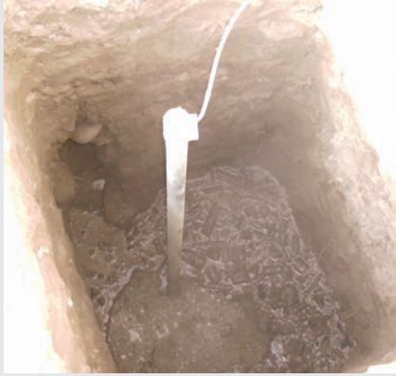
Fig. d: Wire from copper plate passing through GI pipe
