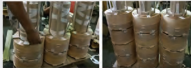
Fig. h: Insertion of bundles of primary coil in the core
