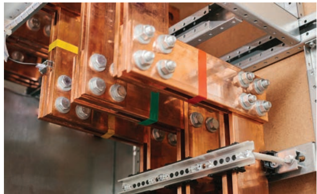
Fig. 4.8: Copper busbar
