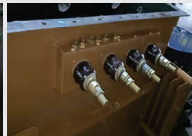
Fig. m: Fitting low voltage bushing on the transformer
