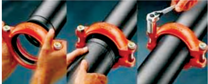
Fig. 5.26: Grooved joint
